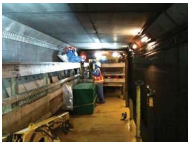
Crew working on one of two specially-designed flatbed cars.
